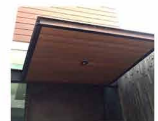
02 SOFFIT MATERIAL - METAL PANEL
