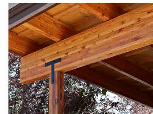
01 GLUED LAMINATED TIMBLER BEAM
